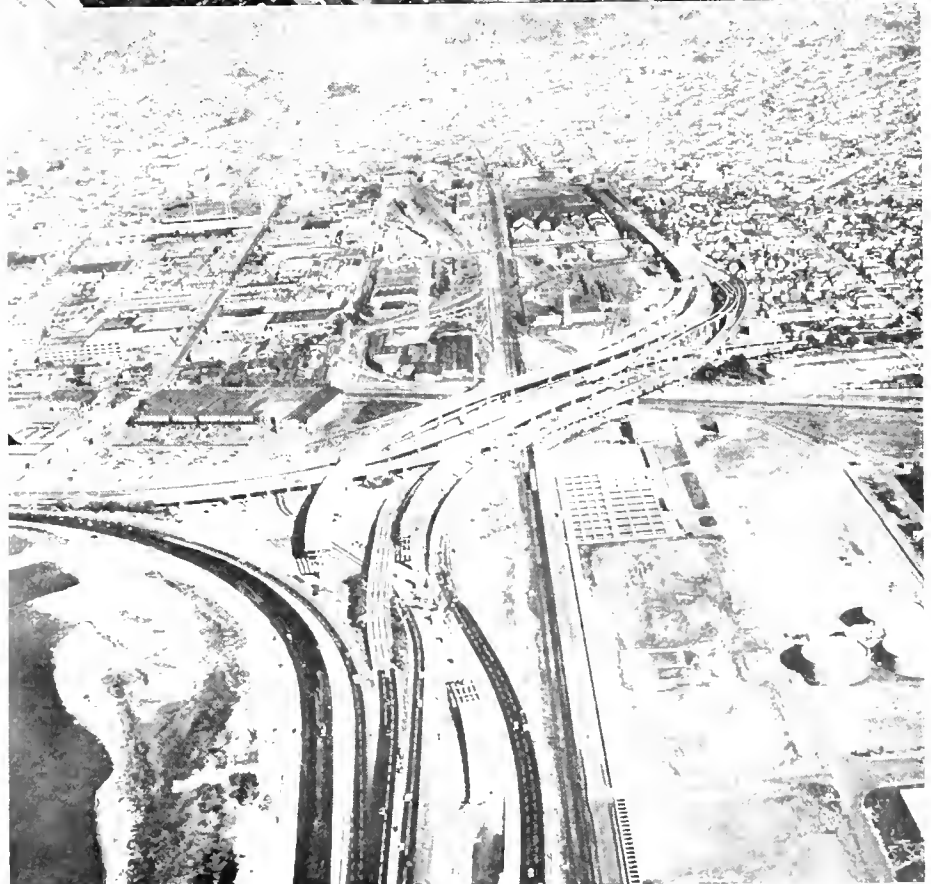
UPPER—Construction operations on additions to the distribution structure looking westerly toward the approach to the San Francisco-Oakland Bay Bridge. The dual two-lane roadways in the lower left of the picture are detours which have been constructed on temporary timber trestles. LOWER—View of construction operations on East Bay Distribution Structure looking east toward MacArthur Boulevard.
